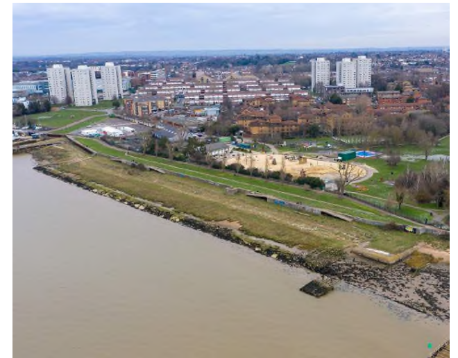
Grays Riverside and Beach Existing
